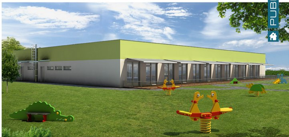
Kungöta, under construction
